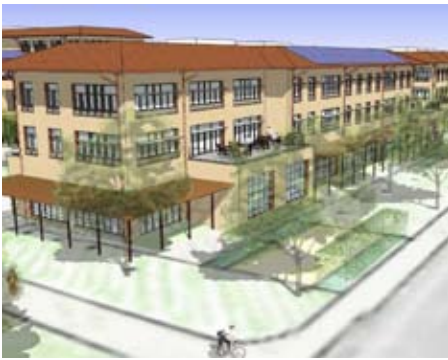
RED TILES WILL COVER ROOFS ONLY PART WAY TO MAXIMIZE ENERGY EFFICIENCY
